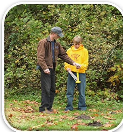
Jake Kvistad working with the Excavator to prepare the site for the installation.
