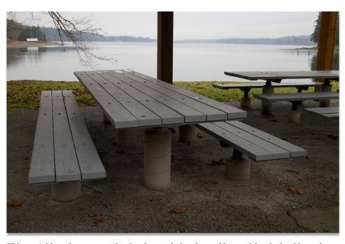
This year's big maintenance project involves replacing the steel bases of the picnic tables and benches under the shelters at the beach park with more more weather/marine resistant concrete, as the old metal bases were corroding through and failing. The work should be complete before spring.
